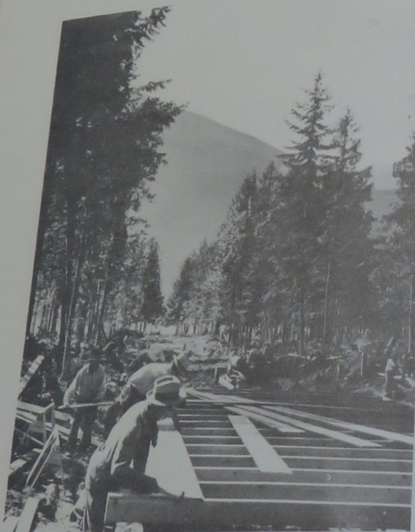
Clearing and laying foundations, New Denver, B. C.
