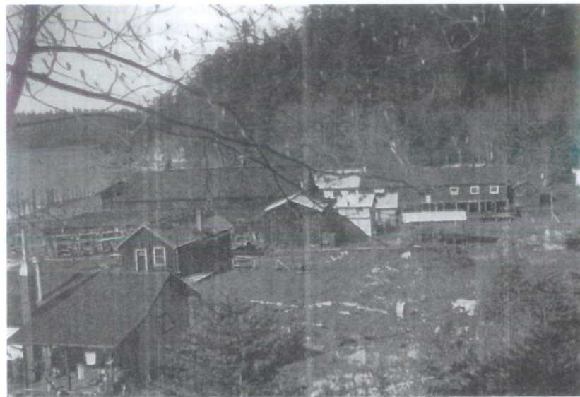
Part of the residential and working space of the Japanese when they were in residence on Newcastle Island. See the series of pilings to the left that were once the supports to one of the large saltery sheds.
