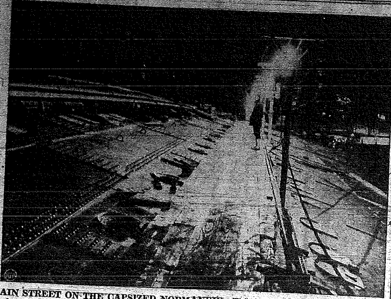
MAIN STREET ON THE CAPSIZED NORMANDIE —This isn't a sidewalk along a metal-surfaced street, but rather a lamp-lit board runway on the side of the U.S.S. Lafayette (ex-Normandie), built to aid in salvage operations of the capsized liner in New York.
