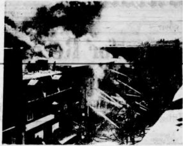
Firemen play ten streams on Montreal fire from short range despite possibility of explosion. Fifteen families were helped to safety from two-alarm fire in downtown district which swept through three buildings with damage estimated at $200,000. Twenty-two other streams of water were played on flames from different angles to keep the fire from spreading. Restaurant and silk-manufacturing firms were demolished.
