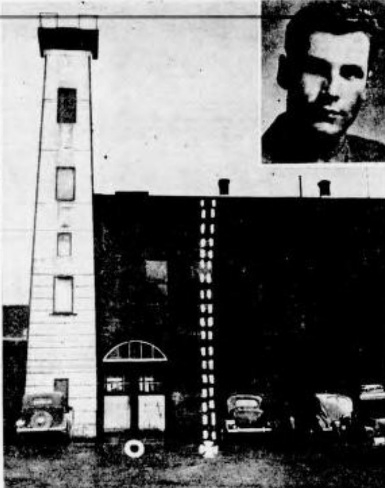
SHOWN above is the rear wall of the city fire hall where a 30-foot antenna ladder slipped during routine drills yesterday morning, causing fatal injuries to fireman Leonard Harper, 24, 722 Russell Street, above, and serious injuries to Chief of Police J. A. McNeilan who was passing nearby. Harper died in the Royal Jubilee Hospital on leave after the accident. Chief McNeilan is in St. Joseph's Hospital suffering from a fracture of the pelvis and four vertebrae and a ruptured kidney. Details in the above photograph show the position in which the ladder was standing before it slipped.
