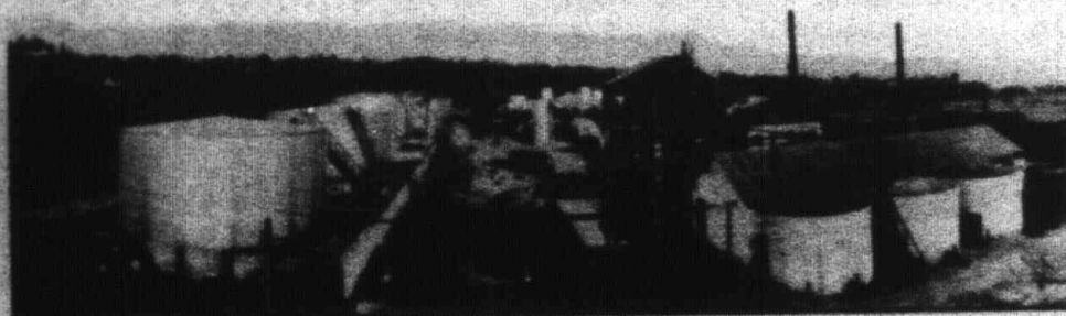
"HOME" REFINERY, NORTH VANCOUVER
